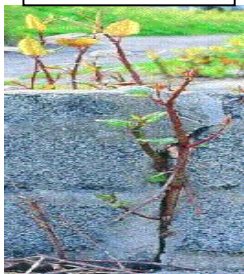
Penetrating a dry, stone wall
