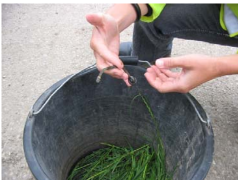
Environmental experts carefully remove reptiles found underneath the tiles
